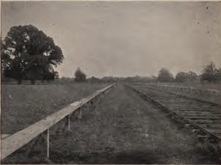
Fig. 77.—View of the track used in my experiments. The machine was run along the steel railway which was 9 feet gauge, and was prevented from rising by the wooden track which was 35 feet gauge.
